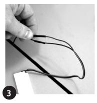
Push into slot – use adhesive for permanent installation.
