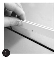
Make 6mm (0.24") slot to required length (25mm/0.98" minimum depth). Bring through power feed from one end of the slot base and solder connections.
