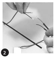
Use heat shrink tube to cover solder joints.
