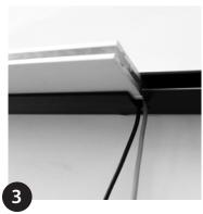
The PVC Channel can be notch cut to allow a cable exit.
